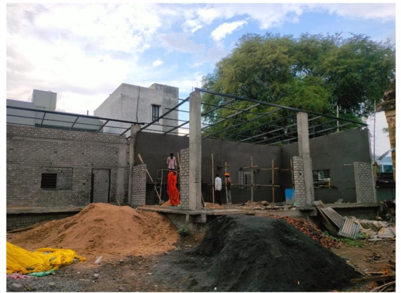
WORK IN PROGRESS
